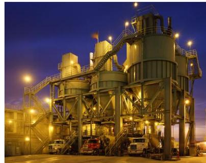
Mitsubishi Cement is proposing modifications to its existing import cement facility located on Pier F at 1150 Pier F Avenue. The facility receives bulk cement and cement-like materials (including Portland cement, blast furnace slag, pozzolans, and fly ash) via bulk cargo vessels at Berth F208. The product is stored in a warehouse and loading silos. It is then loaded onto customer trucks via three truck loading racks and transported to local and regional concrete batch plants.
